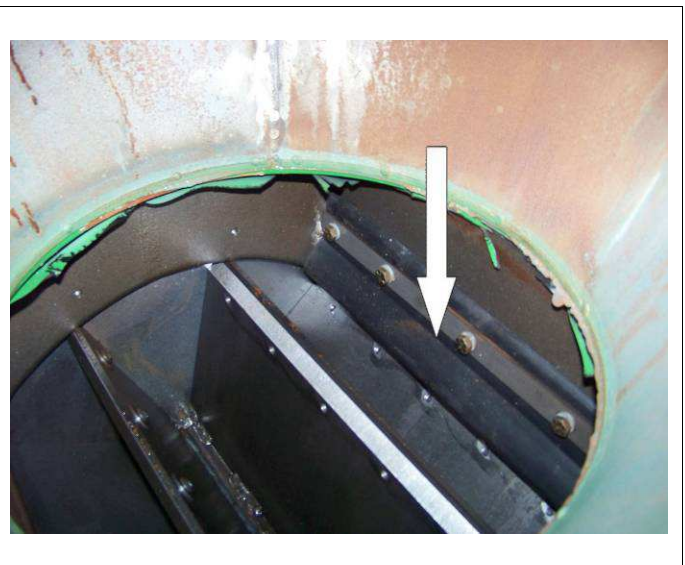
Fig. 5-30 Check Wiper Blade Through The Access Door
