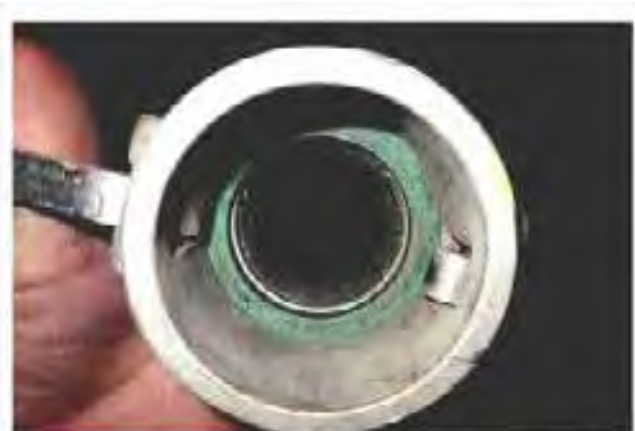
FIG. 18 GASKET SEAL (TYPICAL)
