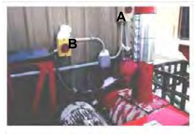
FIG. 3 POWER DISCONNECTS:
